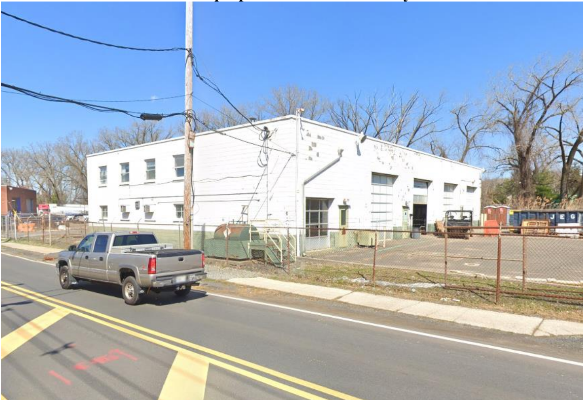
Photo 2: Existing building and utility connection. Utility pole to remain and underground electric connection will be run to the proposed building
