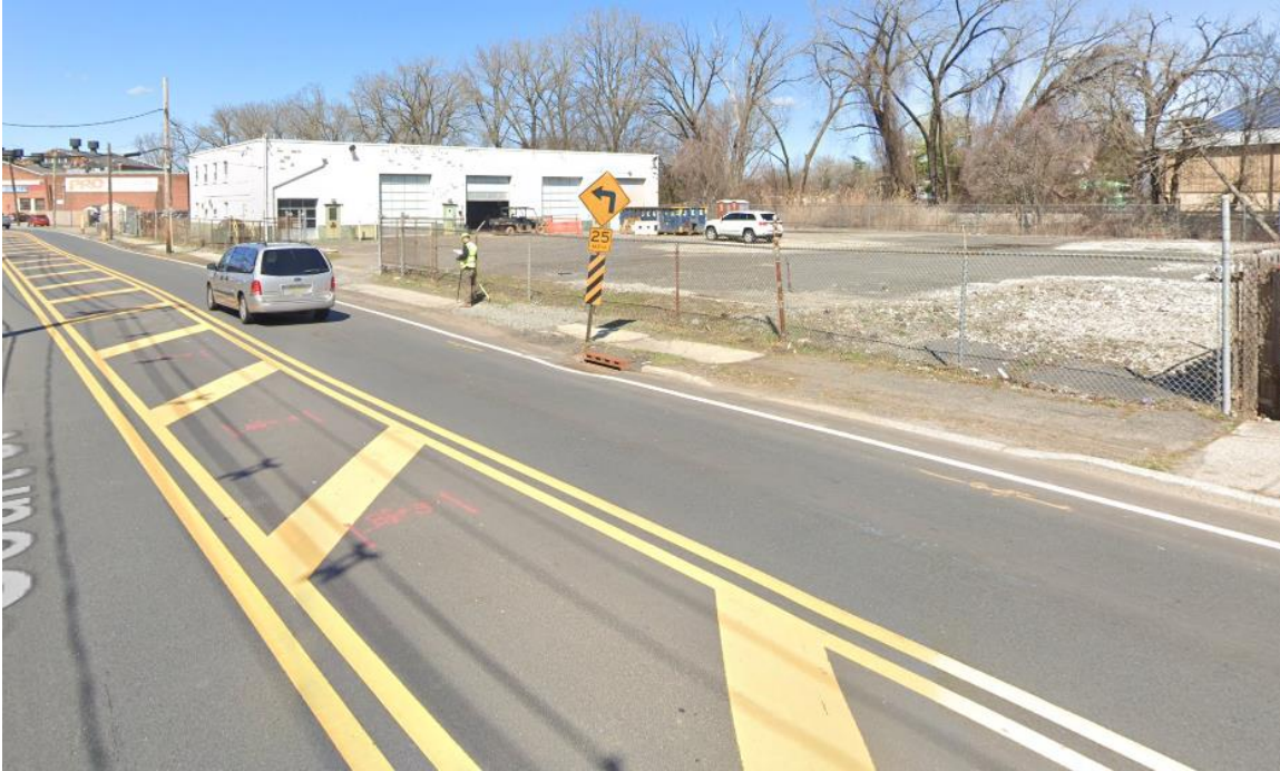
Photo 1: Southwest corner of the existing site along West Fort Lee Road. Location of the proposed southern driveway.
